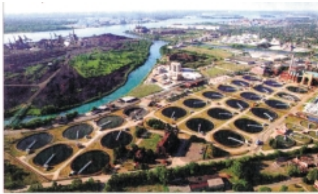
An aerial view of the waste water treatment plant in Detroit.
